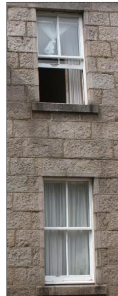
Repair of sash & case windows can often be much cheaper than replacement
