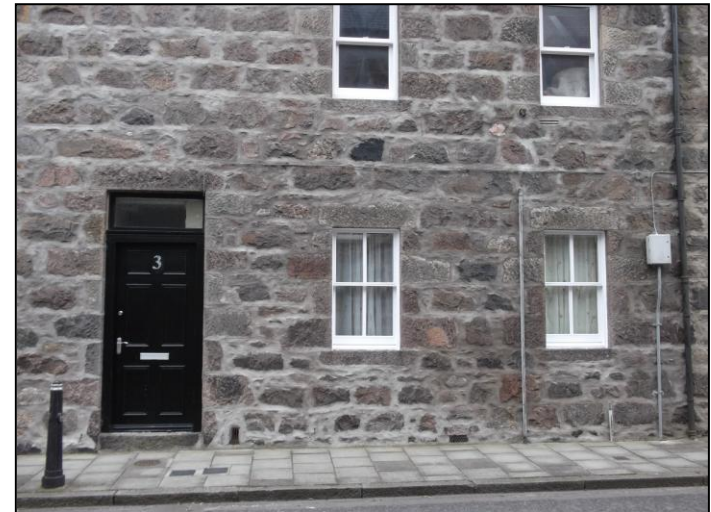
Replacement windows will generally require to be white
