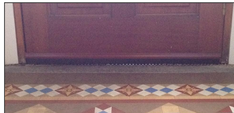
Draught-proofing strips can be easily applied to interior side of external door
